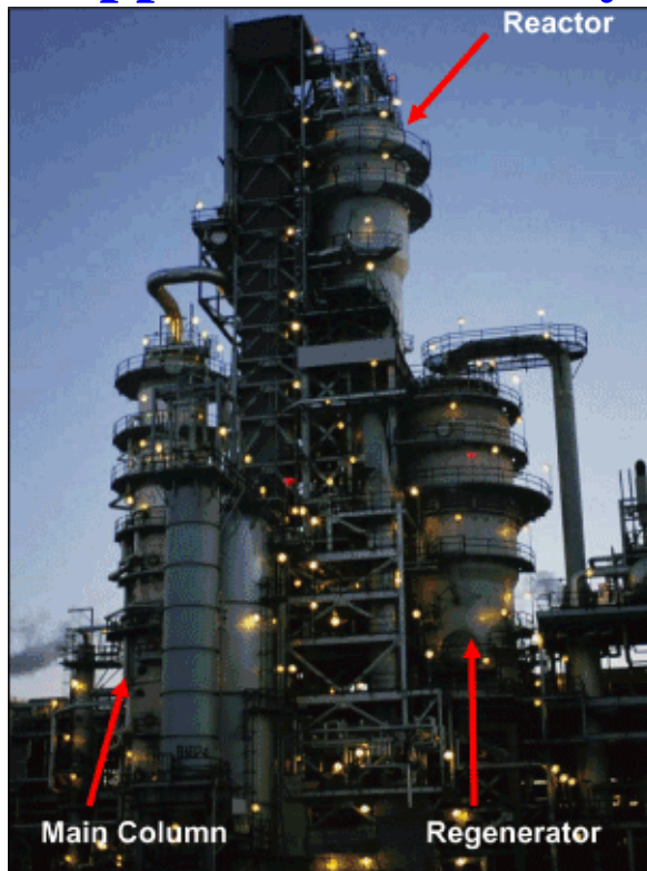
A typical fluid catalytic cracking unit in a petroleum refinery
